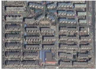
Assess building stock and infrastructure at a localized level
